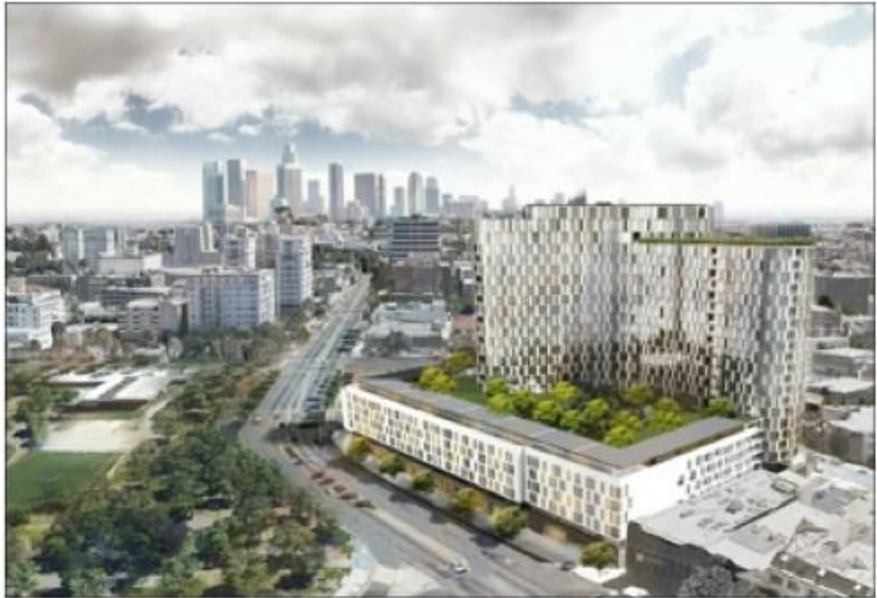
2900 Wilshire 644 Units Jamison Services
