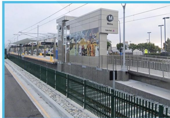
Metro K Line | Crenshaw and Slauson Station
