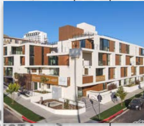
REEVES CONDOMINIUMS 1415 S Reeves St
