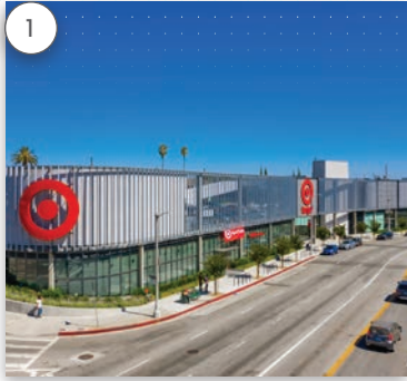
MID-WILSHIRE SHOPPING CENTER 1302-1342 S La Brea Ave
