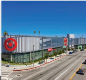
MID-WILSHIRE SHOPPING CENTER 1302-1342 S La Brea Ave
