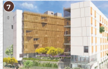
7 ROSA'S PLACE 501 E 5TH ST 98 Units Currently Under Construction
