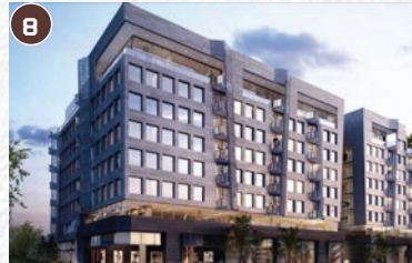
8 409-411 E 5TH ST 409-411 E 5TH ST 150-Unit Proposed Apartment Project
